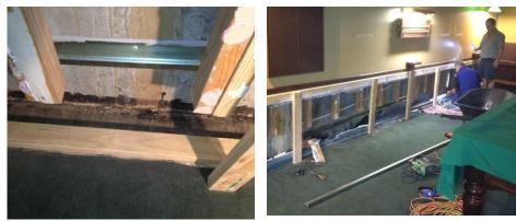
Problem walls often need water to be managed to an exit point. Duel strategy of using the channel to create a fall to exit point, plus floor level 'water stop'...
