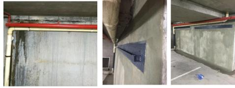
Common problem of water getting through the cold joint flowing down walls and leaving slat deposits can be managed. First apply a Negative Tanking treatment to the joint (Contec C1). Install Drip Channel under joint with masonry fastener, secure with polyurethane and membrane protect surface.
