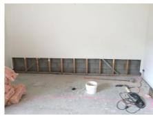
Moisture ruins stud walls effecting the floor coverings.. Apply a Negative Tanking treatment, Use Drip channels as a 'water stop' and means for evaporation or exit channel.
