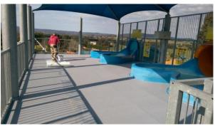
Install a trafficable waterproofing membrane system incorporating MICROL with chopped strand fibreglass. Two coats to achieve the dry film thickness.
