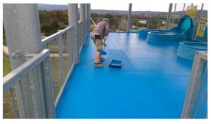
Apply a chemical resistant coating of chlorinated rubber paint to withstand the substances in the water. Swiftvulc – Dolphin Blue Chlorinated Rubber, two coats.
