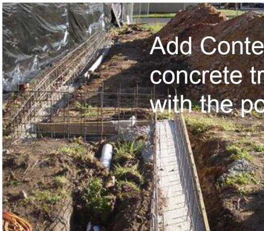
Trench with reinforcement mesh
