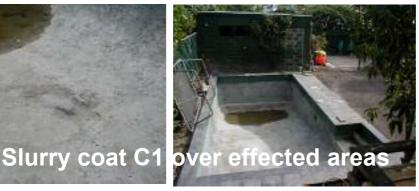
Adding C1 to the crack repair, treats the concrete
