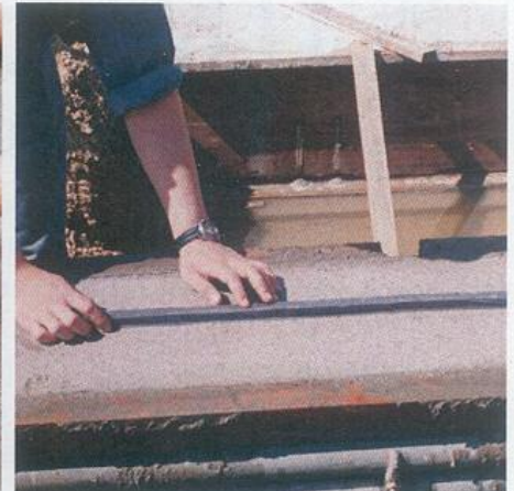
PLACE KUNISEAL ON JOINT AND PRESS IN PLACE.
