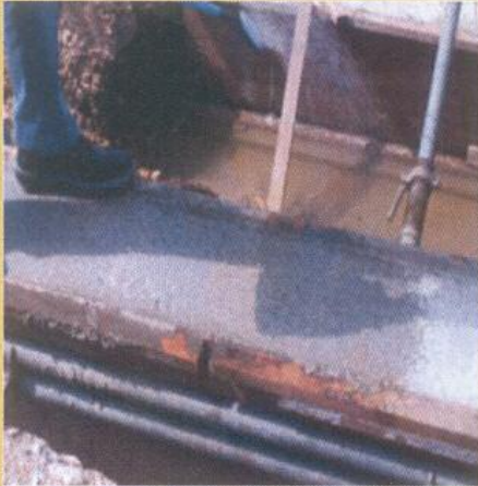
BRUSH OFF DIRT AND WET CONCRETE JOINT.
