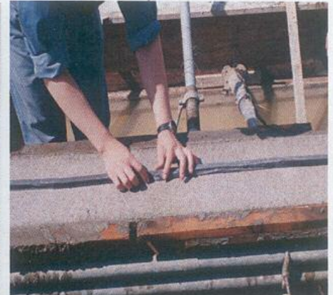
CONNECT TWO PIECES BY END-BUTT JOINING.
