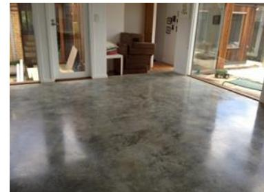
**Burnishing is used for maintenance, rejuvenating and removing mechanical or chemical damage.**
