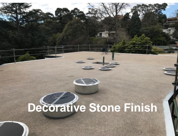
New roof covered with reinforced waterproofing membrane
