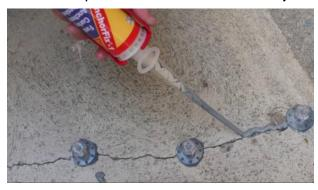
Draw the mixed epoxy (Sikadur 52) inside the syringe (30cc), and mount the syringe into the pedestal. Inject epoxy via the pedestal until there is flow from the adjacent pedestal or until the epoxy stops flowing. Attach the rubber bands to apply a constant pressure if
