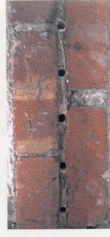
Mortar & bricks saturated with DPC Cream
