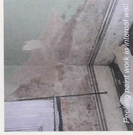
Rising damp shown in internal walls
