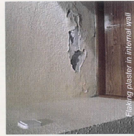
Rising damp shown in internal walls
