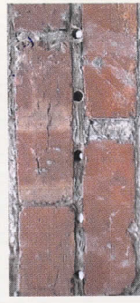
DPC Cream starts penetration
