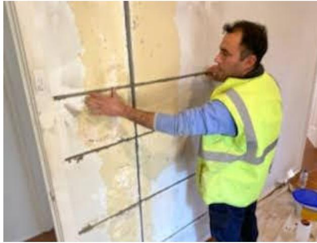
Open horizontal mortar to fit **Helitie Bars** on the vertical and horizontal positions
