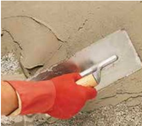
Application of Planiseal 88 by trowel
