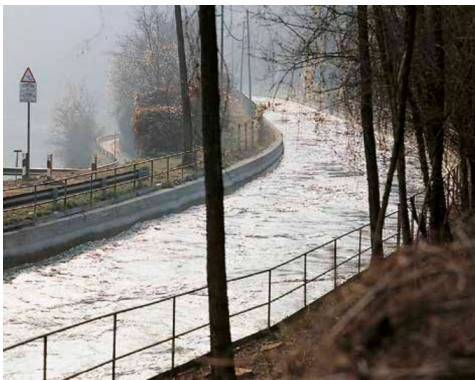
Bertini hydroelectric canal - Como - Italy. Surfaces treated with Planiseal 88
