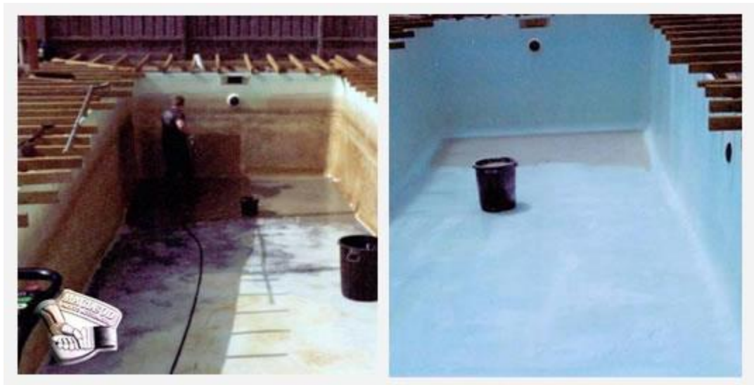
Before and after painting with Macleod's Swiftvulc Chlorinated Rubber.
