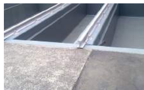
Solutions for Secondary Containment Areas. Page 40
