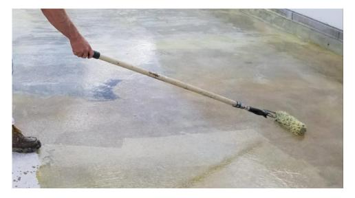
**APPLICATION**: Apply with brush, roller or spray. Keep adding until the surface is no longer absorbent. **Do not allow to pond**. Use prior to membrane system dust-proofer or sealer
